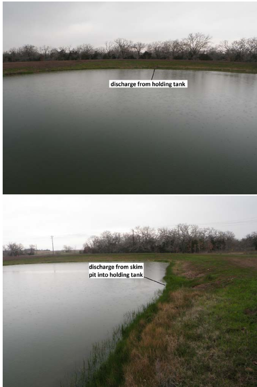
Figure 2. Southwest Muldoon Field Battery 1 Holding Tank on March 5, 2014. Photo by David Buzan, Atkins, at 16:10 CST. Top photo of west side of tank. Bottom photo of east side of tank showing discharge into tank from the skim pits.
